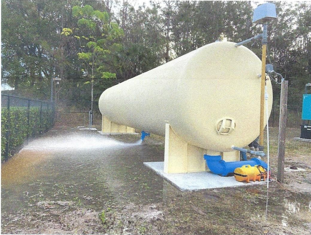
Exterior of Tank
