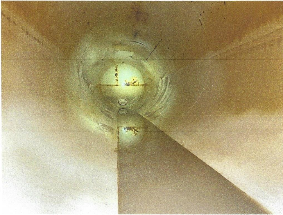
Interior of the tank
