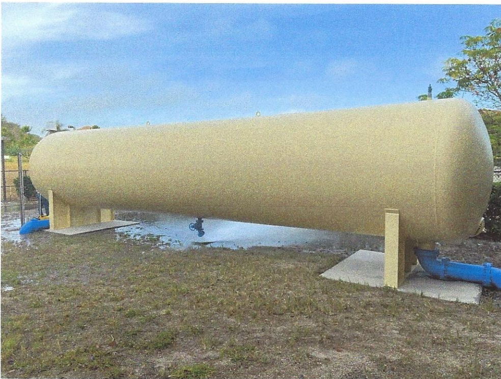
Exterior of Tank
