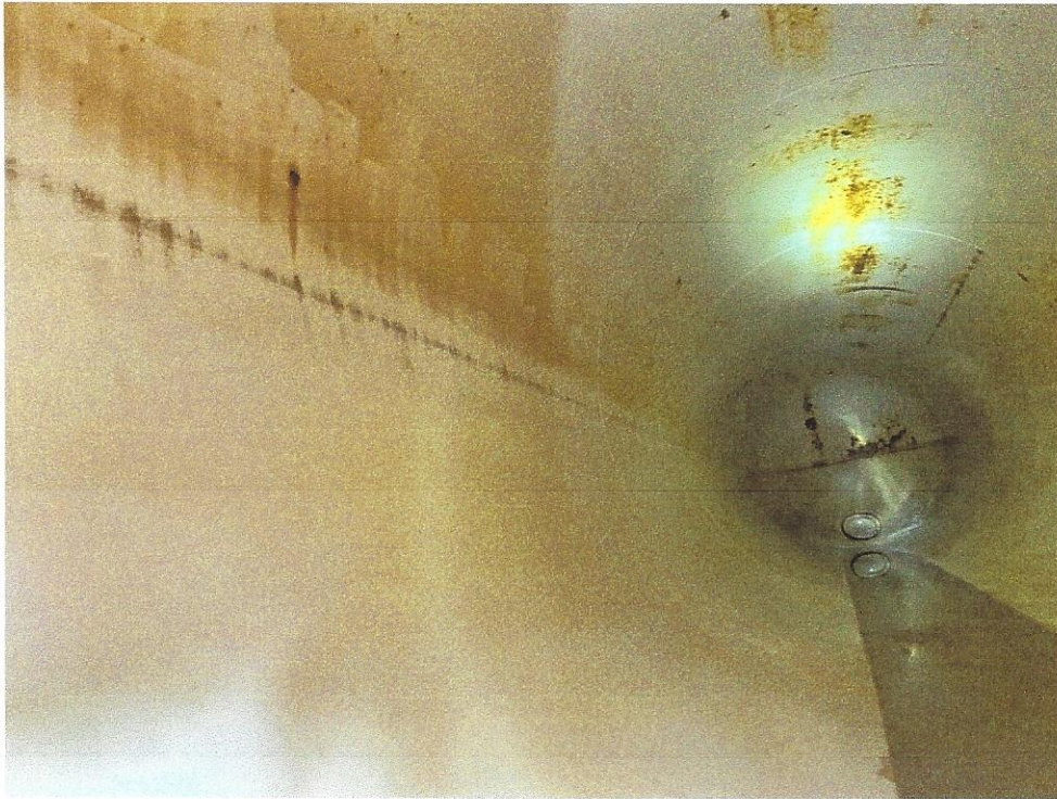
Interior of the Tank
